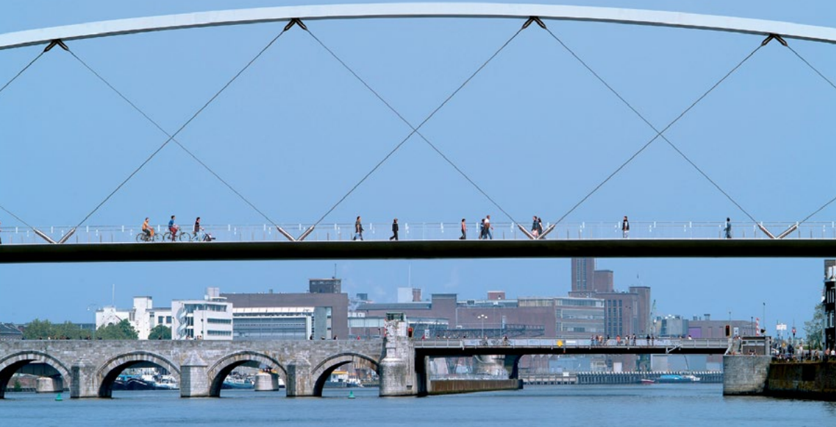
261m-long arch Footbridge to link the new Ceramic district and the old city.
