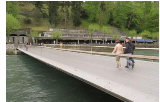
Deformed shape during the use of the footbridge
