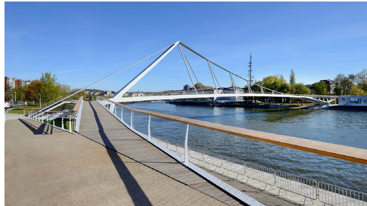
Crossing of the Meuse river in Liege with a width of 7 m and a total length of 294 m, the main span of 163 m is suspended.
