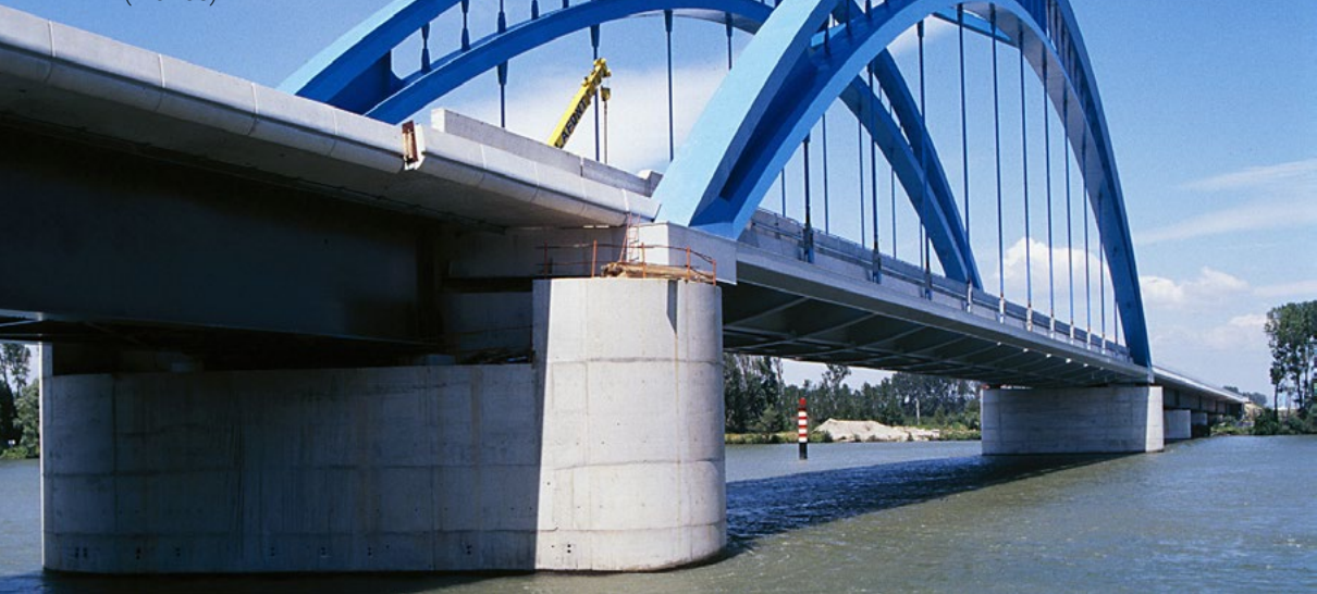
HSR viaduct on the Valence-Marseille high-speed line.
