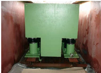
Tuned mass damper (TMD)
