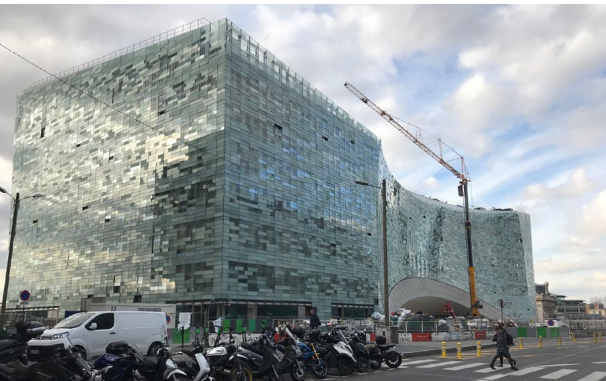
«Le Monde» new headquarters in Paris (total floor area of 23,000 m 2 )
