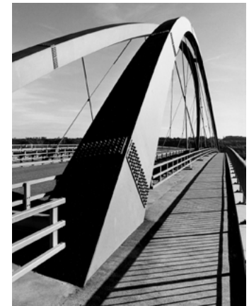
Instability verification without or with very light bracings.
