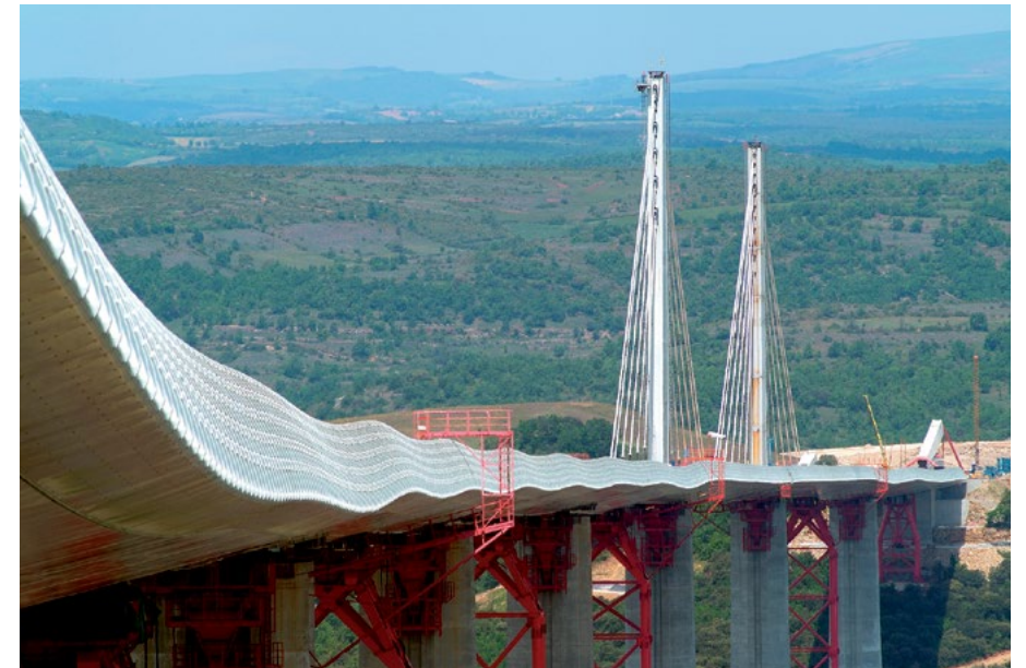
Deformed shape of deck during launching
